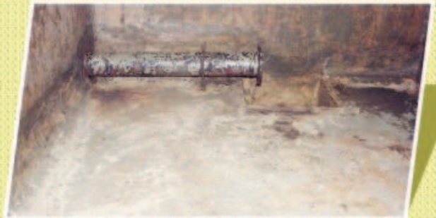
After Cleaned rusted Inlet & surface of tank
