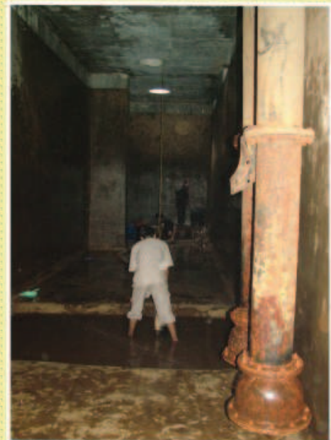
Removed of Sludge & Muddy Water
