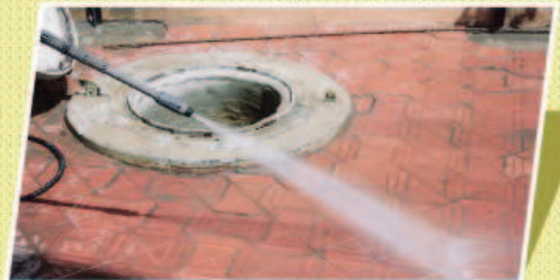
After Cleaning of Tank surface
