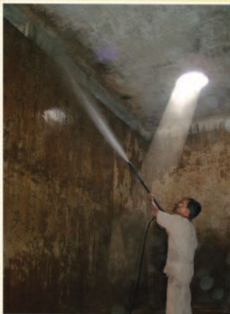
Cleaning of Tank Ceiling & Side Wall
